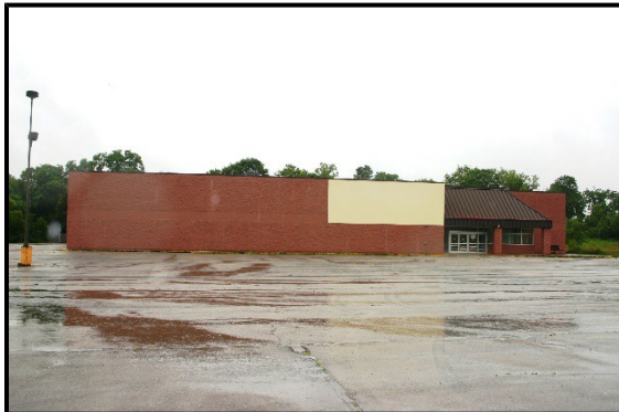
1300 Jefferson Street, Greenfield, OH
